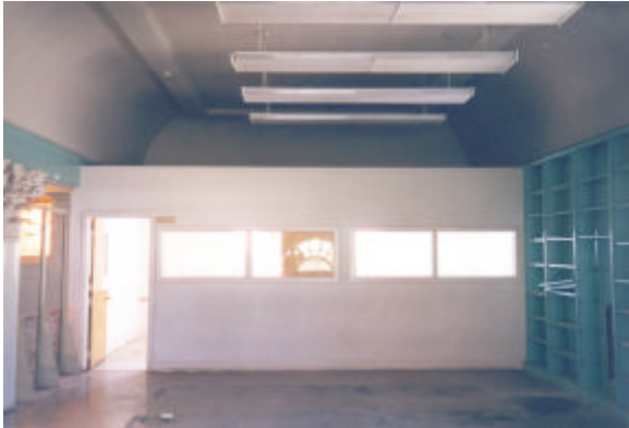
Interior walls like this one, built on the Gallery Level in 1965 to create a second private librarian's office, disrupt the open plan interior and daylighting and should be avoided.
