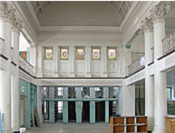
Existing derelict interior.
