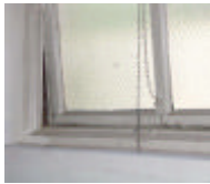
Above: aluminum windows on the East elevation. Left: 1912 wire glass and metal sash.
