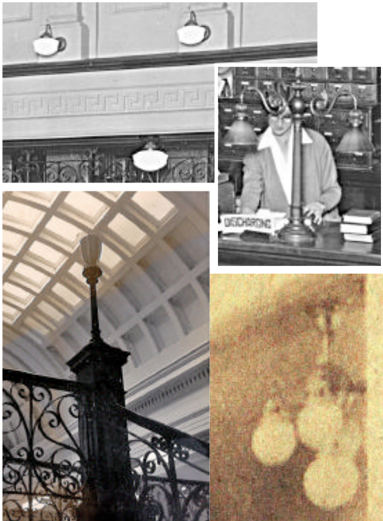
Clockwise from top left: Schoolhouse style; original desk lighting fixture; original globe-style fixture; and balustrade fixture with fluorescent system installed in 1945. Historic photographs courtesy of the Alameda Museum.
