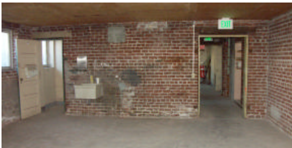
Insulation could be applied to historic exposed brick exterior walls in the basement. Interior walls would remain brick.
