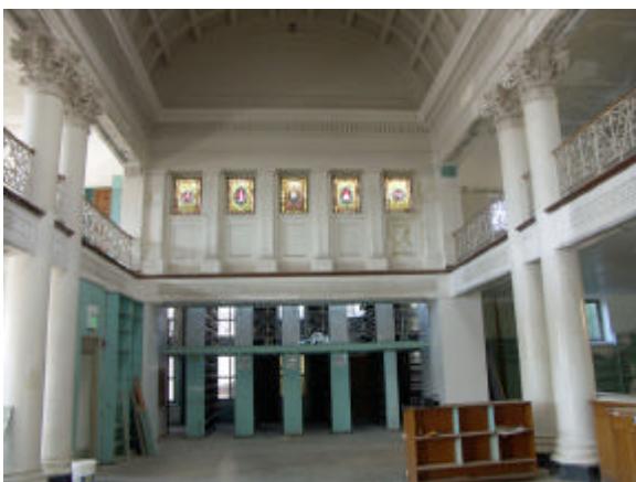
Overall photograph of stacks and relationship to the second floor and atrium.
